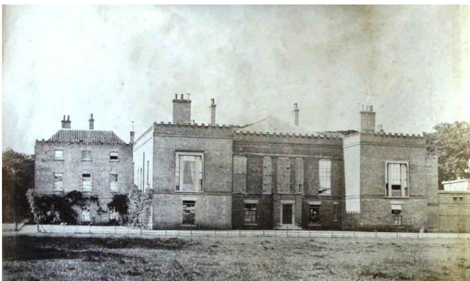
High House at Westacre
