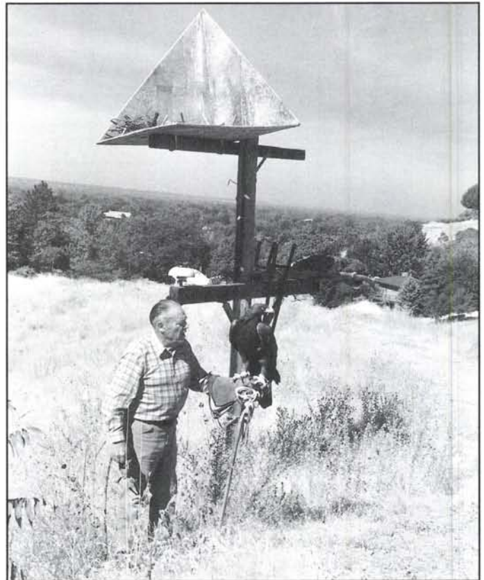
Mock up power pole and nest platform erected by Idaho Power Company for Nelson's work to save eagles from electrocution
