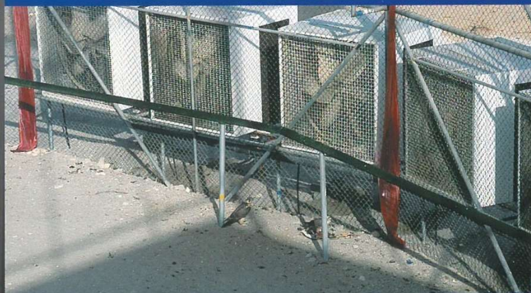
The huge fans that constantly blow water-cooled air into the flight pen.
