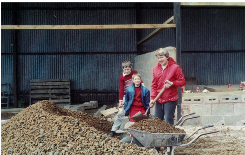
Constructing the Owl Wood aviaries
